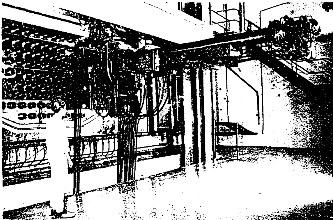
FIGURE 31 Pickering Fuelling Machine
